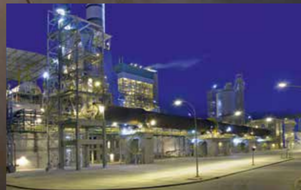
Steuler is exclusive refractory technology partner for lime kilns of Andritz Pulp + Paper. Together we are shaping the future for lime kiln refractory performance.
