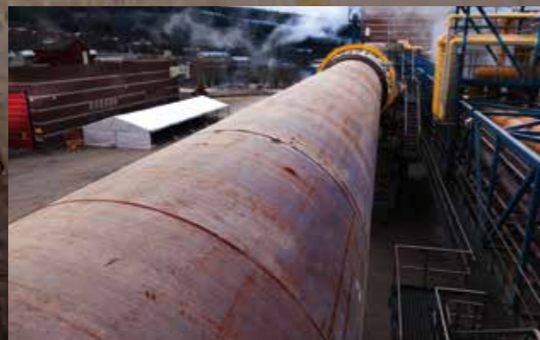
New construction of a lime kiln for a pulp mill capacity upgrade. Inside view of refractory lining can be seen in the background of the picture.
