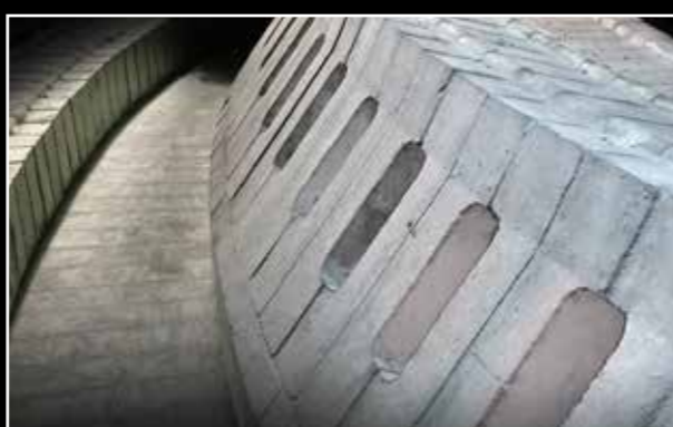
Assembly of gas inlet area with special tongue and groove bricks
