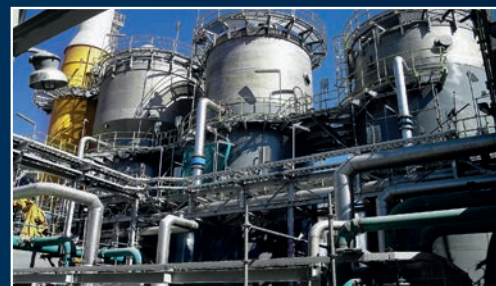
Absorbers, process basins and pipes are e.g. lined with rubber and additional bricks in non-ferrous metal extraction and acid production plants.
