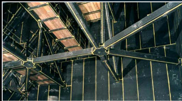
Rubber lining in a flue gas scrubber.
