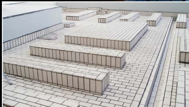
Combined lining system composed of sealing membrane and ceramic tiles in a containment basin.
