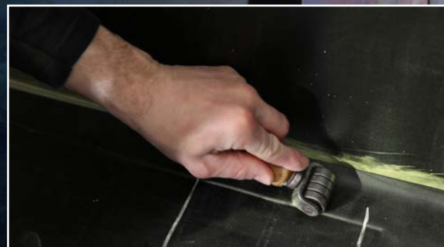
Application of a rubber lining.
