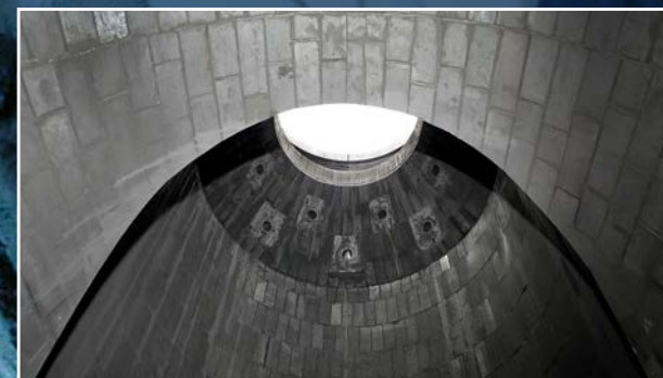
System lining with carbon bricks.
