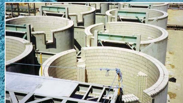
System lining with ceramic bricks.
