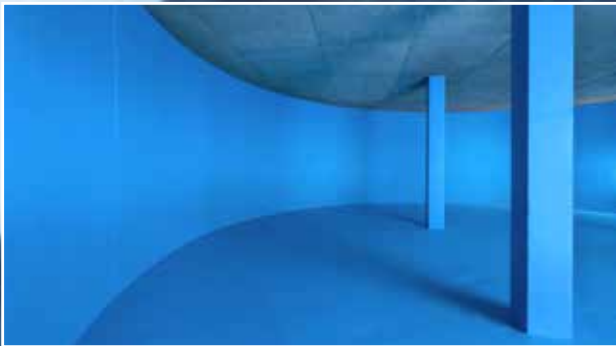
BEKAPLAST AQUA LINING in a drinking water reservoir.
