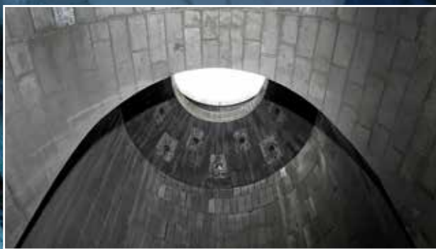
System lining with carbon bricks.
