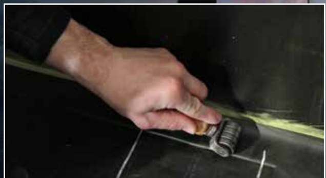
Application of a rubber lining.
