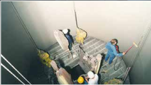
Leak testing of a chimney coating.
