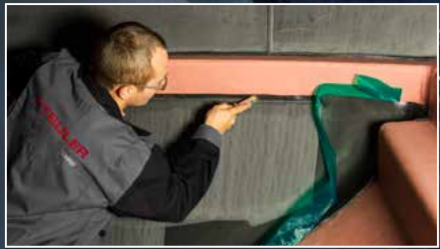
Controlled conditions: Installation of a workshop rubber lining.
